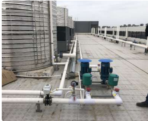
Pipelines for Waste Heat Recovery
